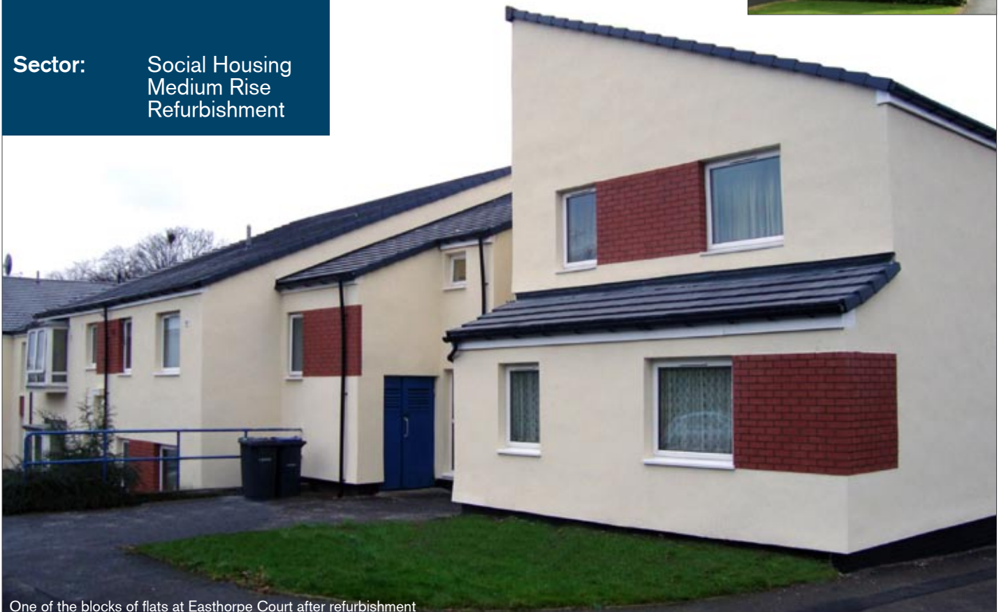
One of the blocks of flats at Easthorpe Court after refurbishment
